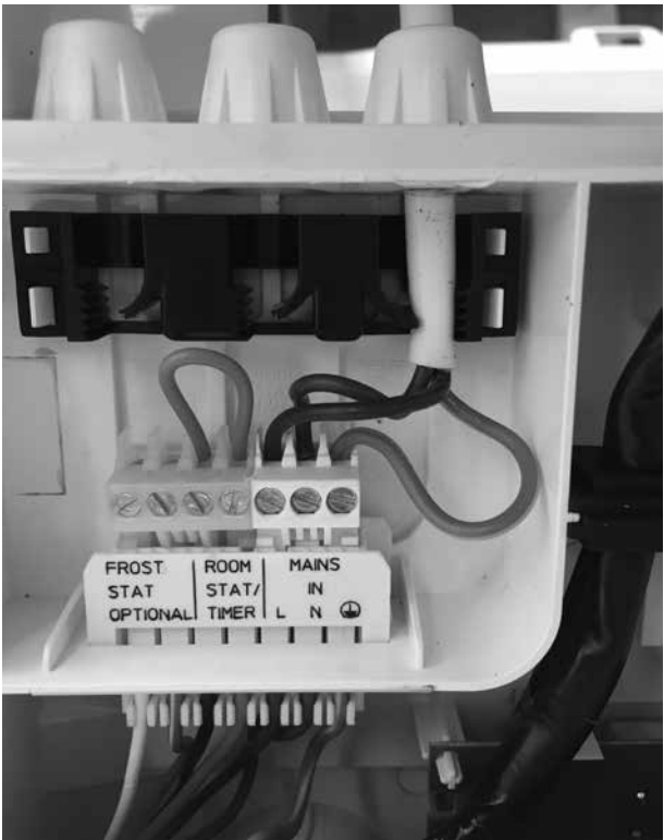
INSTALLER CONNECTIONS (LHS)
